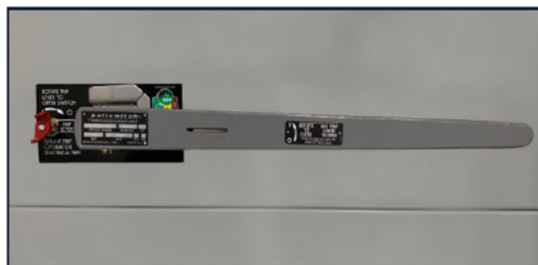
Bolted Pressure Switch (BPS)
