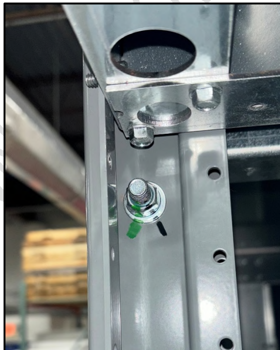
Section to Section Fastener
